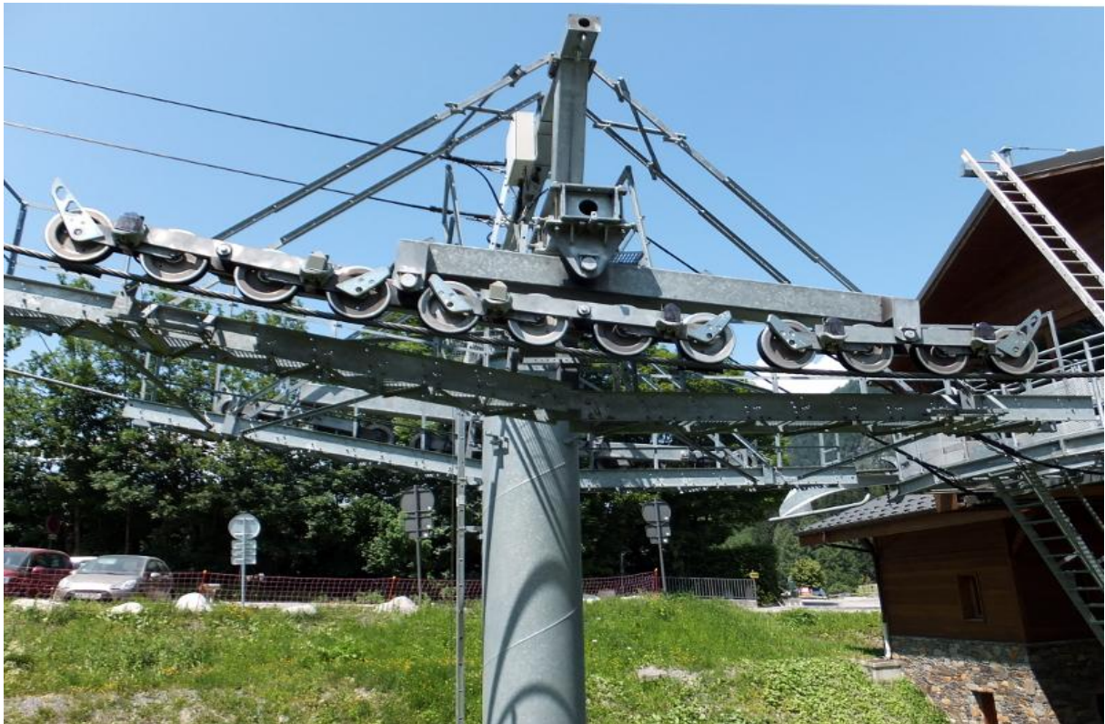
Figure 44 Pylône compression (12C) [31]
