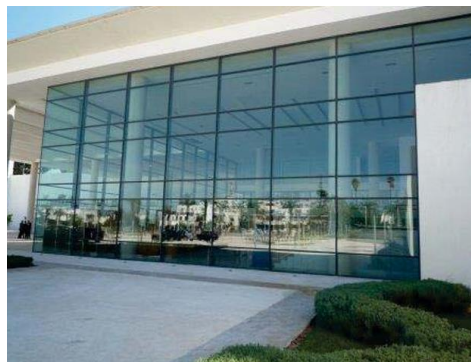
Figure 78 : facade mur rideaux vec
