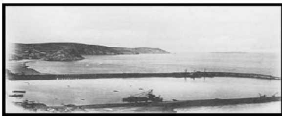
Figure 45: Le port de Beni Saf 47
