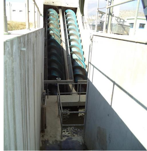
Figure III.04: Photo vis d'Archimède.
