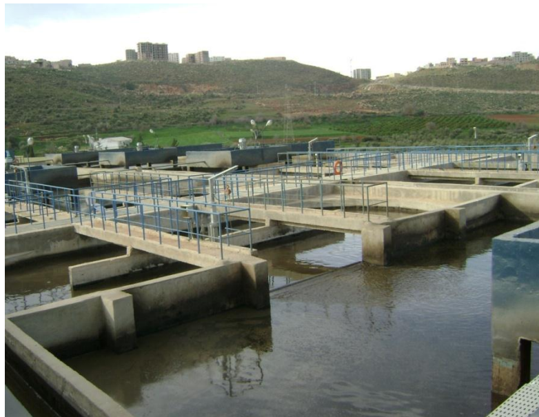
Figure III.9: Photo du bassin de nitrification dénitrification
