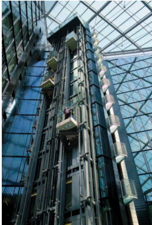
Figure 103: Ascenseur double lift same shaft 93
