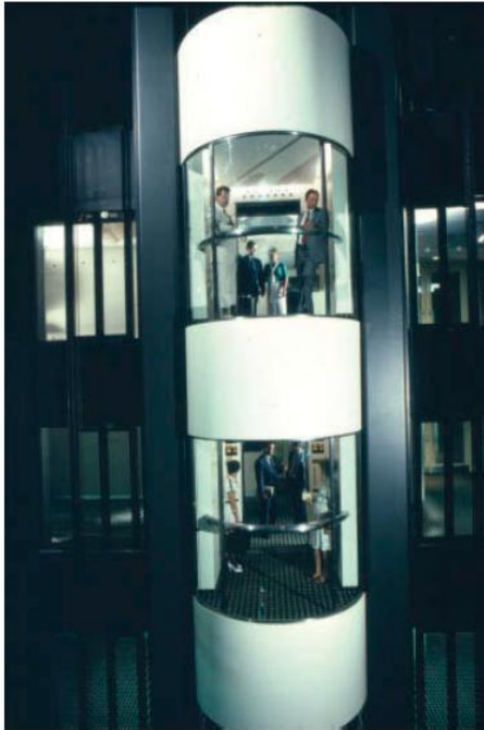
Figure 102: Ascenseur double Deck system 92
