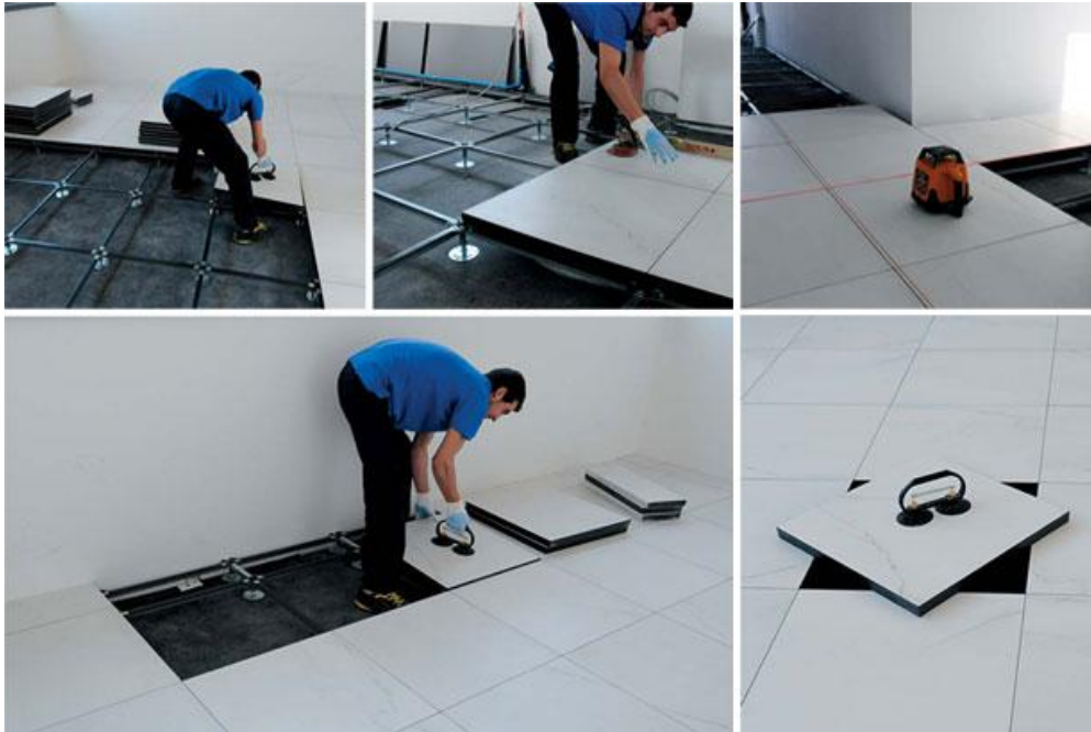
Figure 188: installation d'un plancher technique 150
