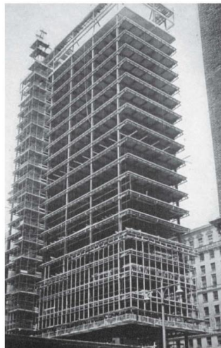
Figure 88: Systeme stick utilisé a Lever House building 77 (Dave Parker, 2013)
