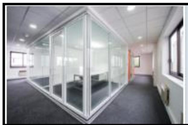
Figure 93: cloison vitré
