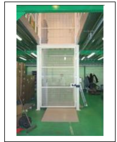
Figure 100: Monte charge industriel
