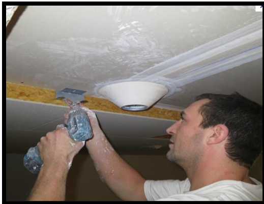
Figure 238 Installation du Dome
