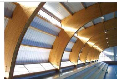
Figure 95: structure lamellé collé
