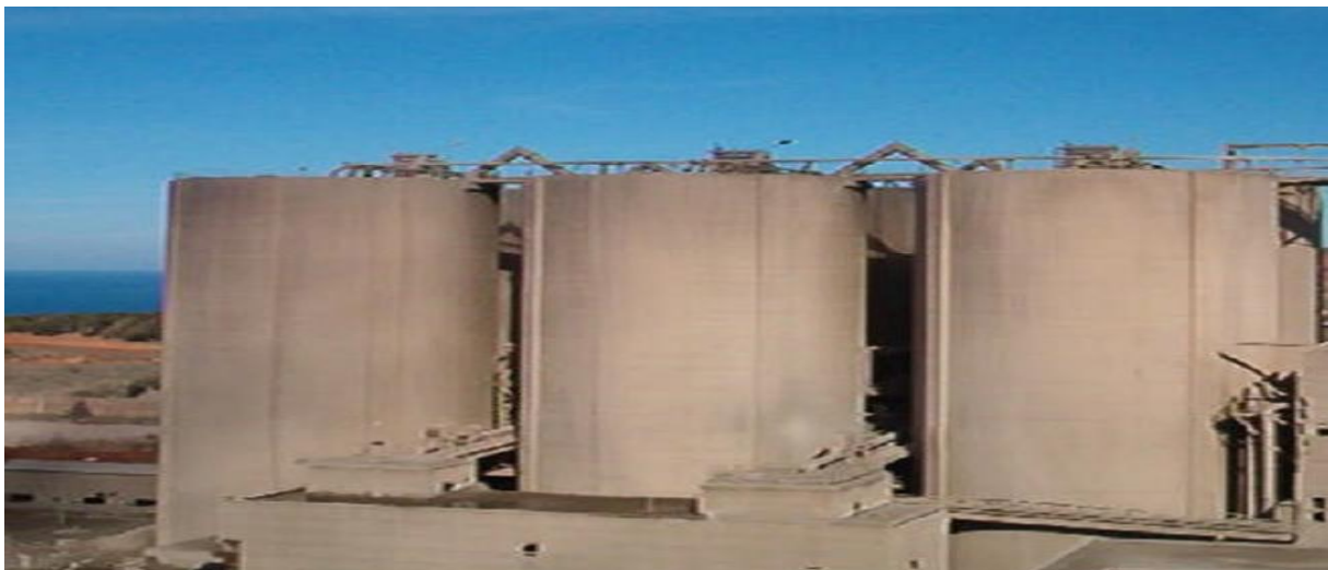
Figure I.17: Silos de stockage de ciment [25]
