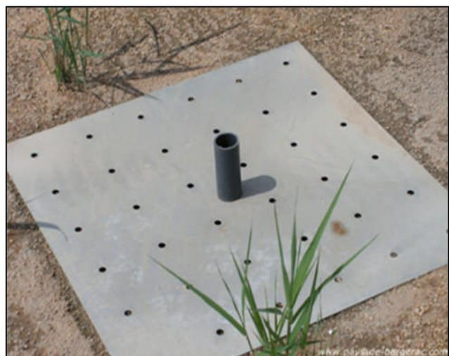
*Figure IV.12: Plaque anti-affouillement.*
