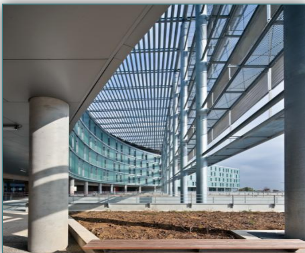
FAÇADE SUD, TERRASSES
