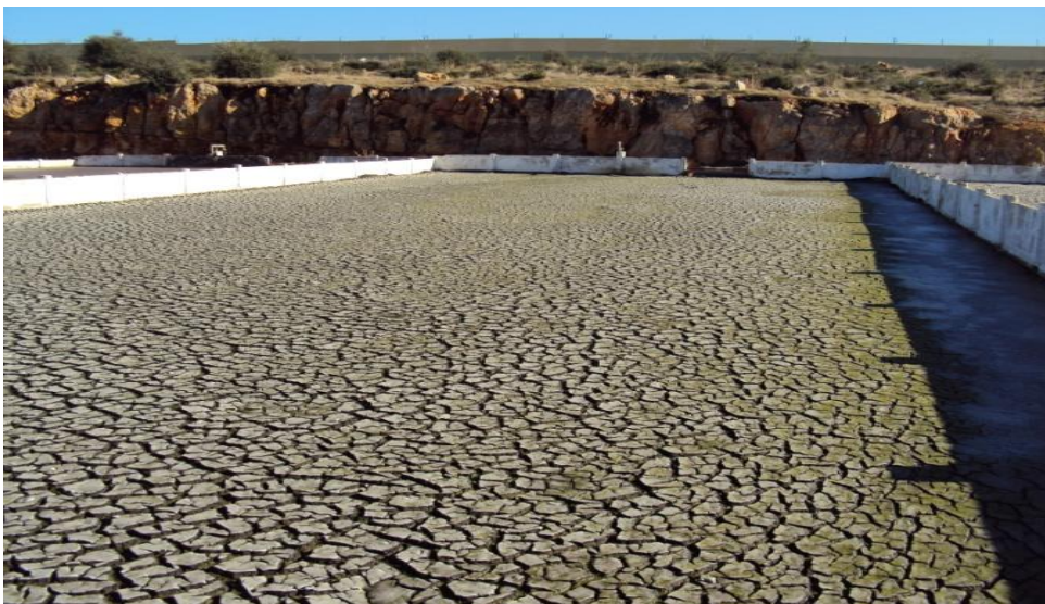
Figure II.12 Lits de séchage [2]
