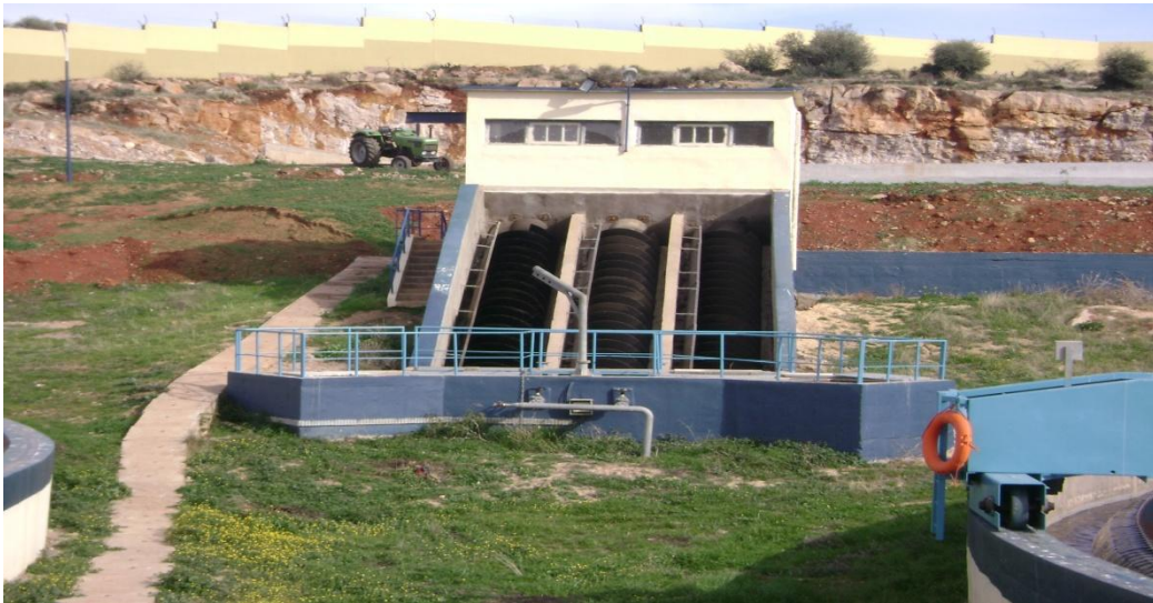
Figure II.9 Vis de recirculation [2]
