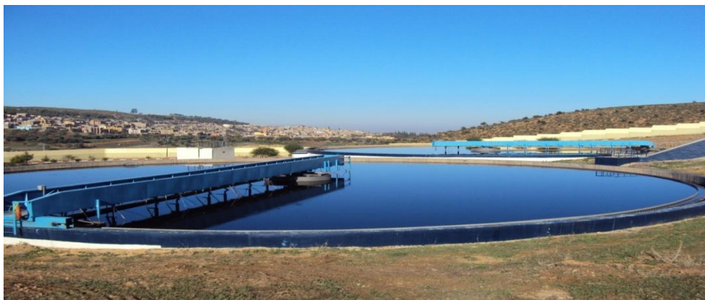
Figure II.7 Clarificateurs [2]
