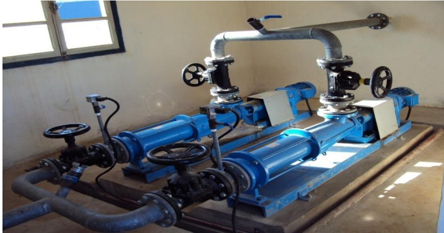
Figure II.11- Pompe de la boue [2]
