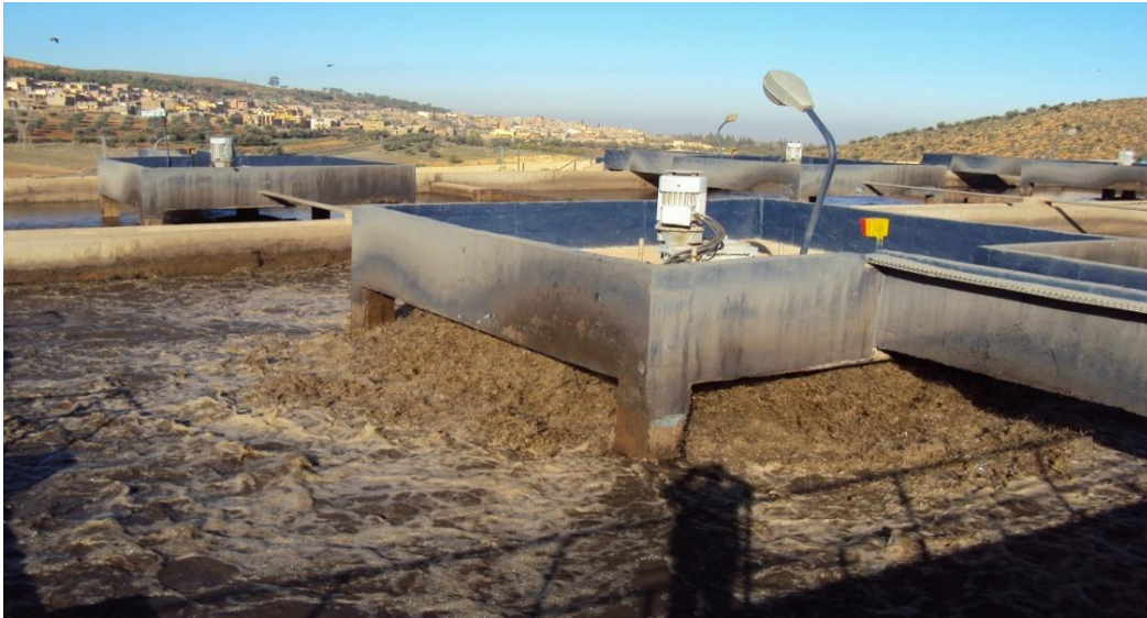
Figure II.6 Bassins d'aérations [2]
