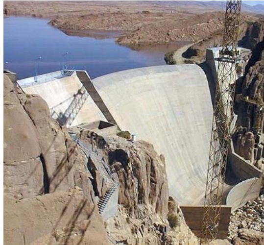
Figure 4.2: Brezina concrete arch dam.
