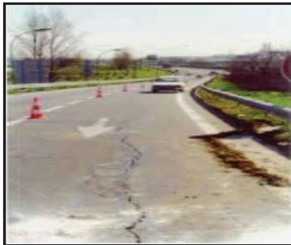
Figure 2.11 Fissuration due au retrait-gonflement (Ferber V., 2005)
