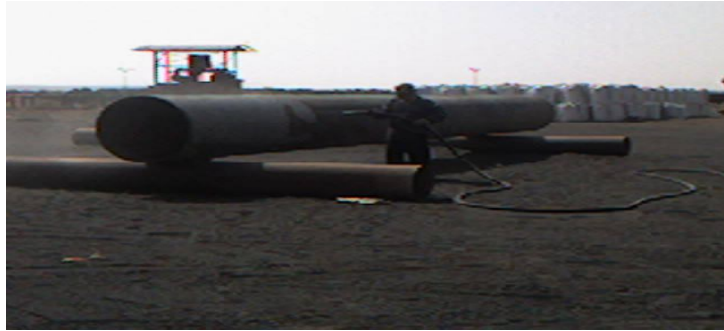
Figure 2.18. Sablage manuel.STT
