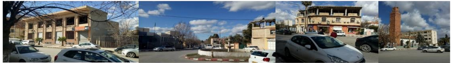
Figure 52: la façade Nord
