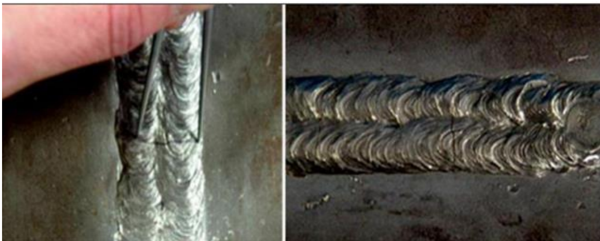
Figure III.7 : La fissure transversale
