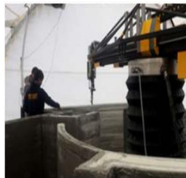
**Figure 1.17: l'impression 3D mobile**
