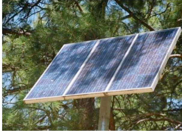
Figure I.6: Partial shading due to trees [43]
