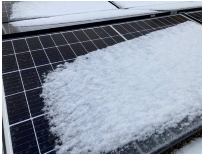
Figure I.8: (a): Solar PV panel covered due to snow [44]
