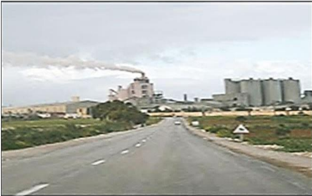
Figure II.8 : Cimenterie de Béni Saf (Photo originale,2016)
