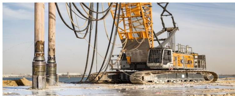
Figure 1.12: LA VIBROFLOTTATION
