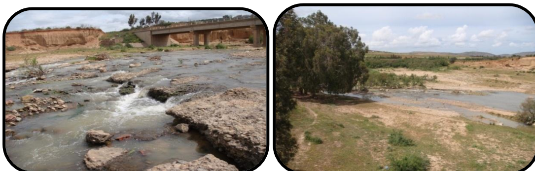
Figure 32 : Photos de la station T.RE
