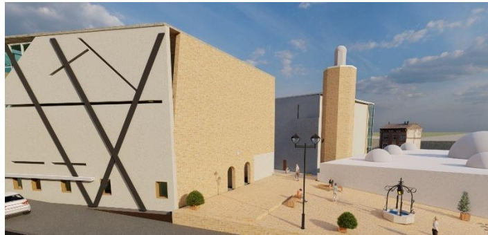
Figure 86: façade du mouçalla
