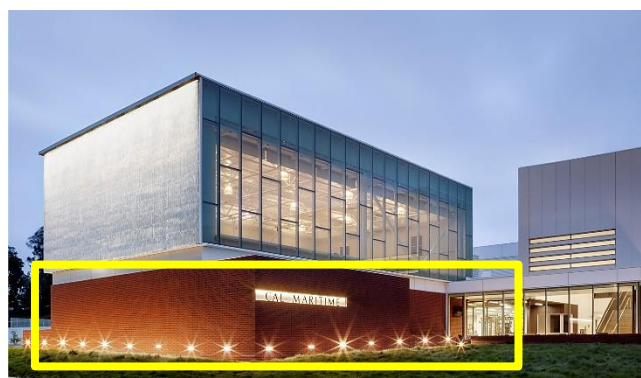
Figure 80 Façade de Cal maritime
