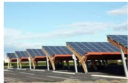
Figure 160 Ombrière photovoltaïque Source : Google image
