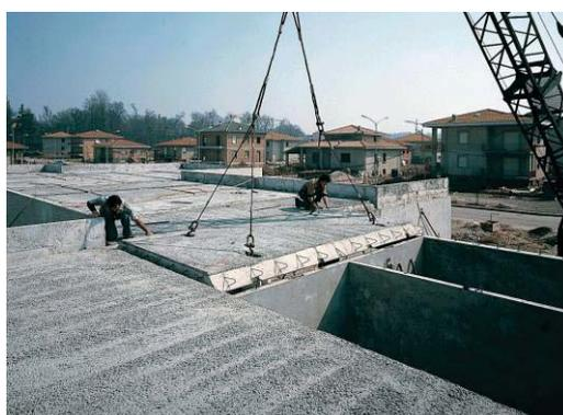
Figure 7: des éléments prefabrication legere
