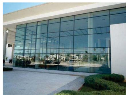
Figure 124 facade mur rideaux vec source(<https://www.sepalumic.com/mur-rideau-vec-vep-aluminium>)
