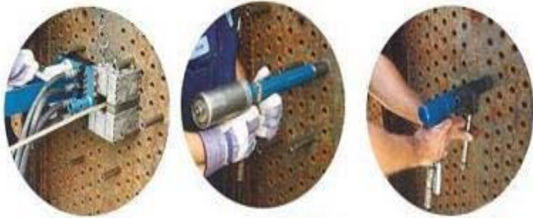
Figure V.4 : Nettoyage des tubes. [3]
