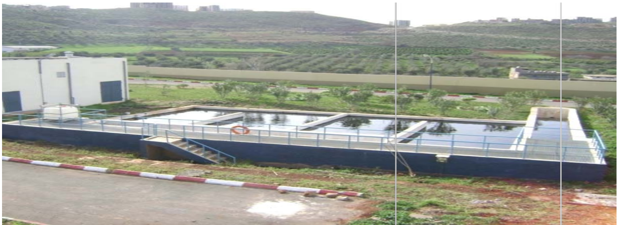
Figure I.12. Bassins de chloration
