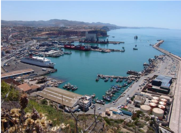
Figure II. 4: Port de Ghazaouet.
