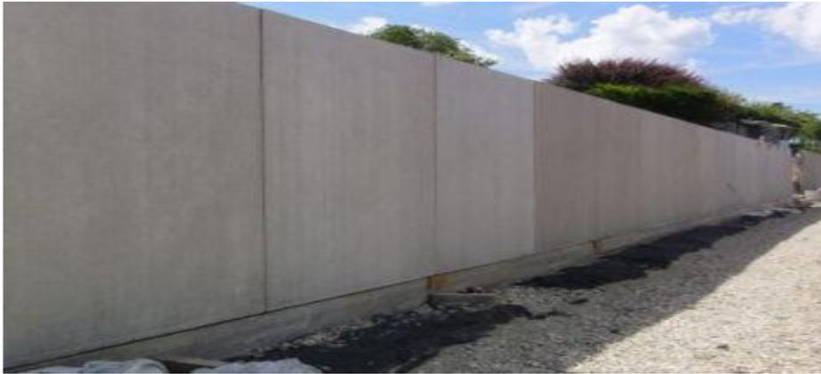
**Figure 27 Mur cantilevers**
