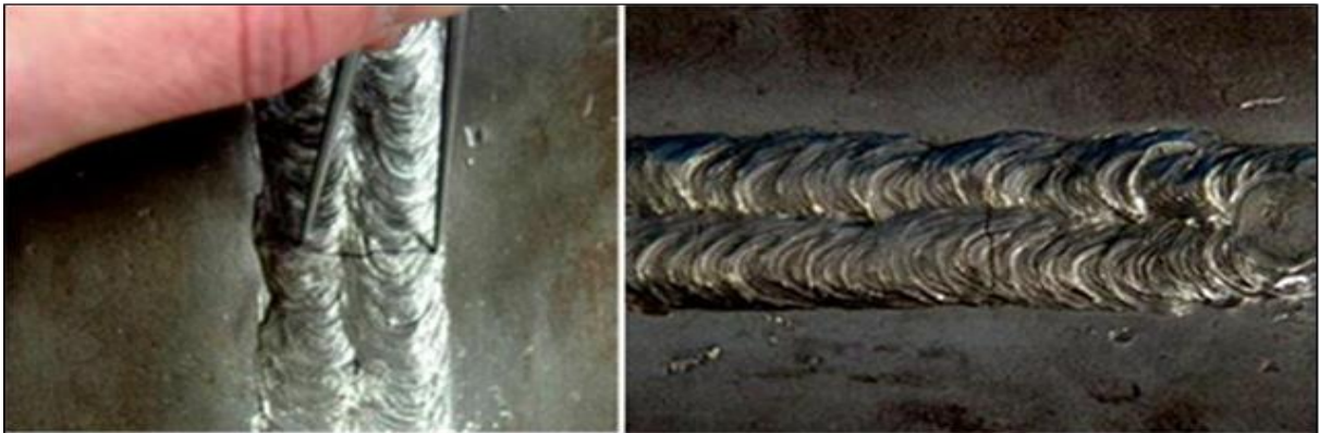
Figure II.2 : La fissure transversale. [11]
