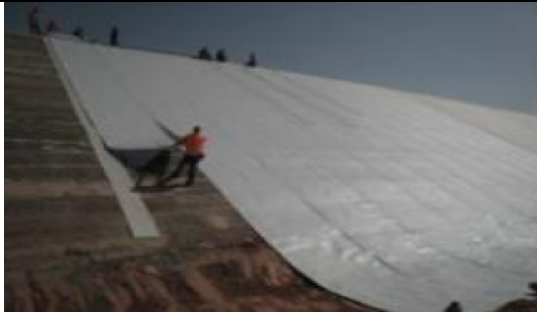
Figure II. 16: Pose d'une geomembrane [25].
