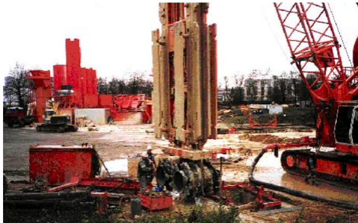
Figure II. 21: Hydrofraise : excavation d'un panneau [28].
