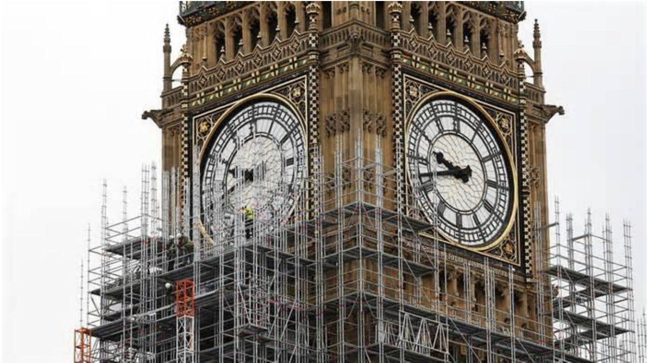
Figure I.2 : restauration de Big Ben
