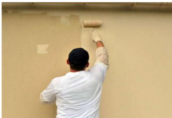
Figure 1.10: application de l'hydrofuge (Alain, 2015)
