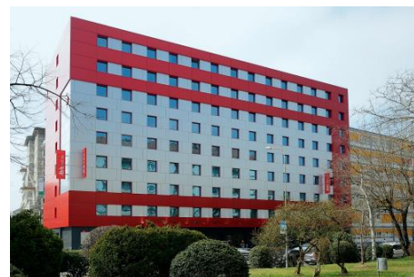
Figure 70: la facade de l'hotel ibis
