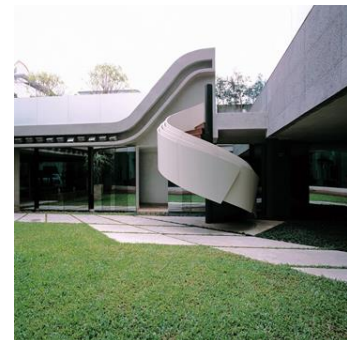
Figure 76: l'escalier de la cour (source: archdaily)
