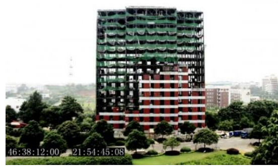
Figure 2: construction de l'hôtel de Changsha source : the architect's newspaper
