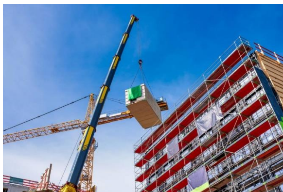
Figure 18: montage des modules pr fabriqu  (source:google image)
