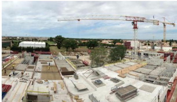
Figure 4: construction in-situ (source : www.sudprefabrication.com )
