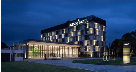
Figure 44: hotel linx (source:archdaily)
