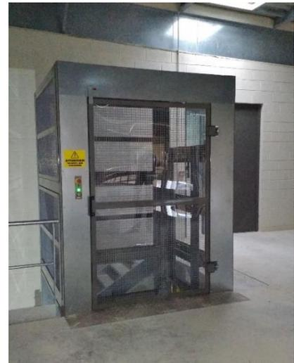
Figure 61: monte charge hydraulique
