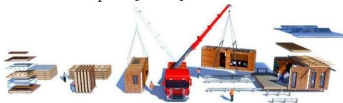
Figure 35 : Installation procedure [BKK16].
