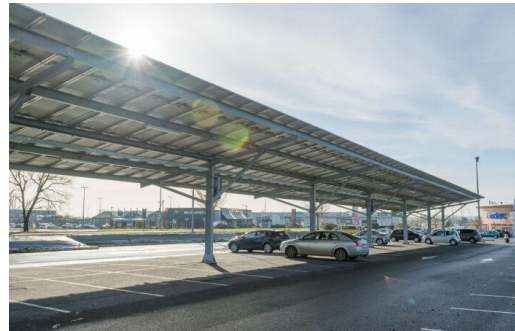
Figure 129: ombrière photovoltaïque Source: google images
