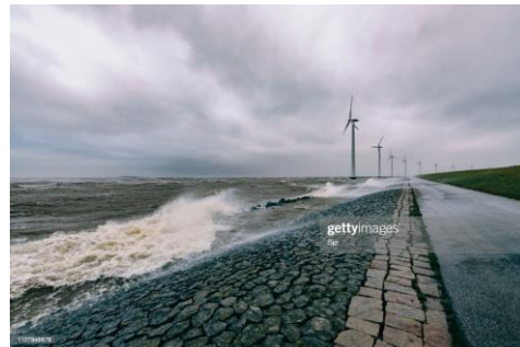
Figure 123: digue de protection Source: google images
