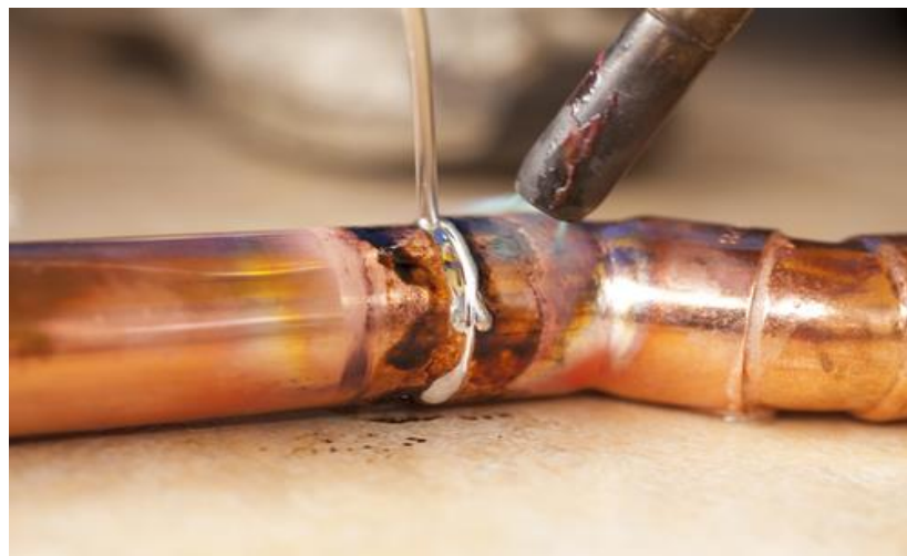
Figure I-11 : la brasure tendre [11].
