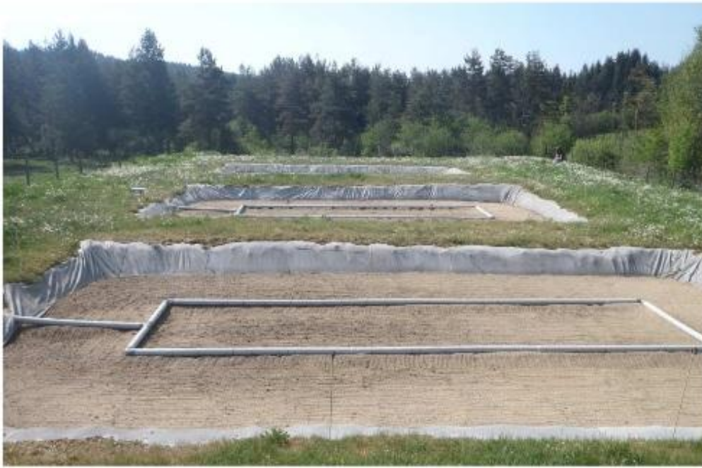
Figure II.11: Bassins d'Infiltration Percolation de Merle-Leignec [28]
