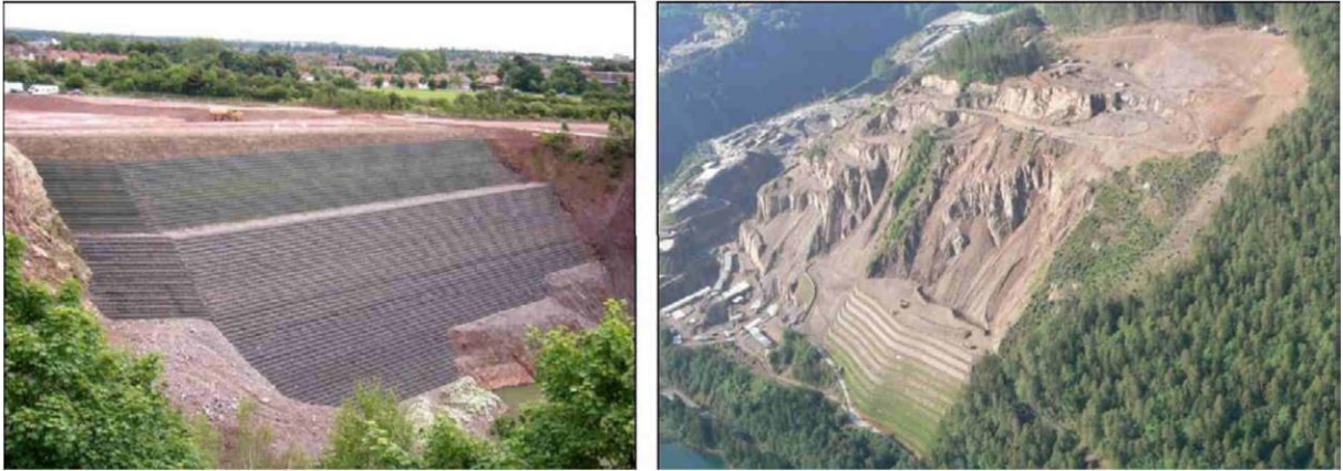
Figure 2.1. Géogrille renforcée raide slopes (google image)
