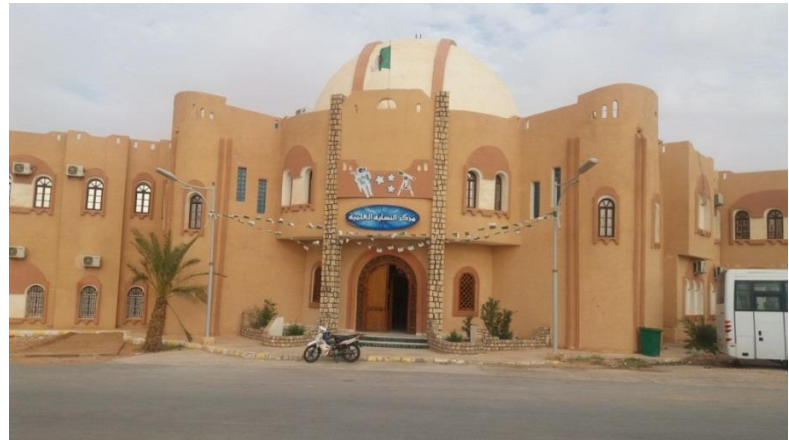
Figure 83 : La façade principale
