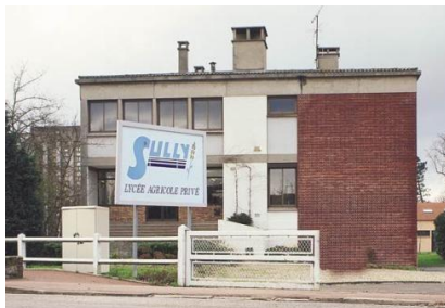
Lycée agricole Sully
