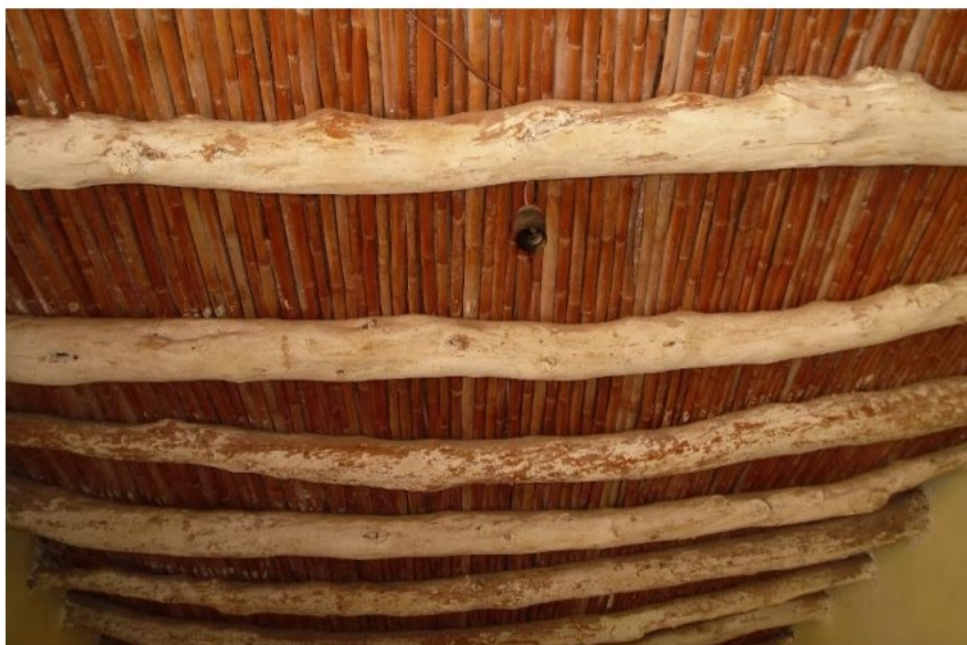
Figure 42: Logs and reeds in a Traras house roof. Source: Authors
