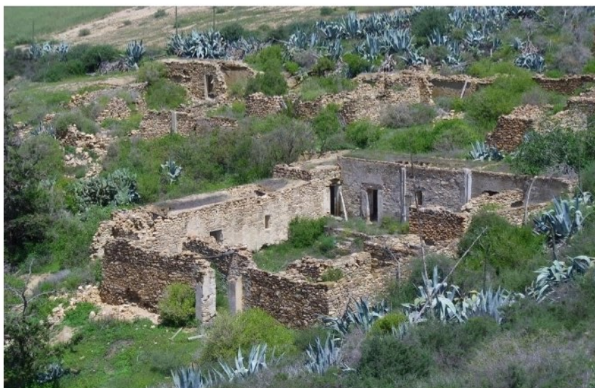
Figure 17: An existing traditional rural house located in the region of Swahlia, Mjiaa village.
