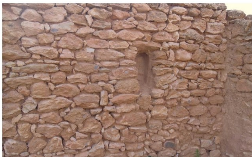
Figure 40: Wall stone ( Tifkart ) masonry bond used in the majority of the Traras Mountains constructions and particularly in the regions of Beni meshal, Jebala, Beni Menir, and Beni Khaled. Source: Authors
