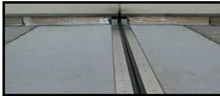
Figure 77 : joint de dilatation.
