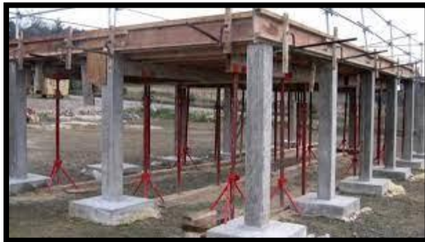
Figure 74: Poteau forme carrée
