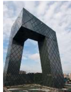
Figure 7 CCTV Headquarters structure en diagrid
