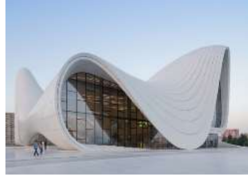
Figure 20 Heydar Aliyev Center / Zaha Hadid Architects
