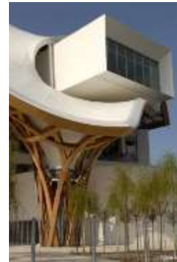
Figure 10 Centre Pompidou Metz Structure en lamellé-collé
