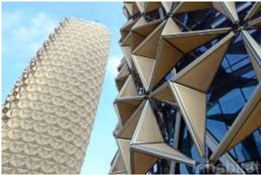
Figure 79 Panneaux amovibles Al Bahar Towers
