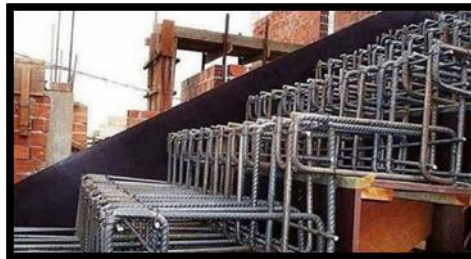
Figure 142: reinforced concrete stairwells:
