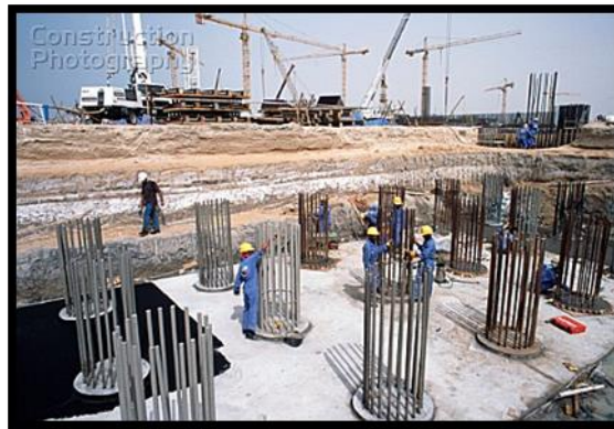
Figure 139: pile foundation:
