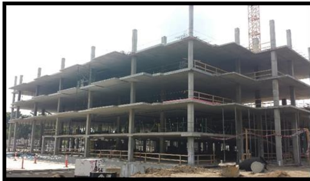
Figure136: skeleton structural system:
