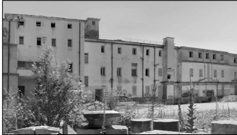
Figure 110. Façade Est, campus Saint-Charles.
