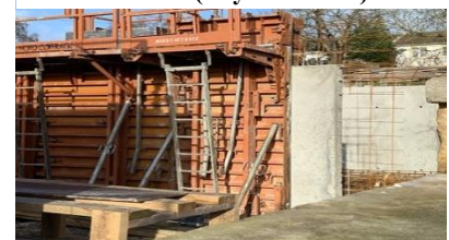
Figure 24: table banche Source : (Asyikine 2013)
