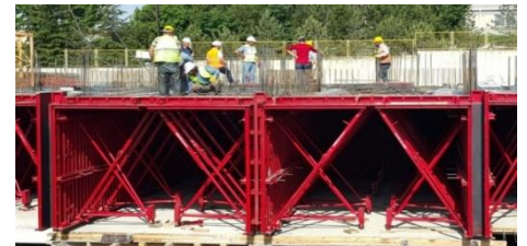
Figure 23: table banche Source : (Asyikine 2013)
