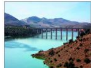
Figure 22: Les barrages Source : www.dta-tlemcen.dz
